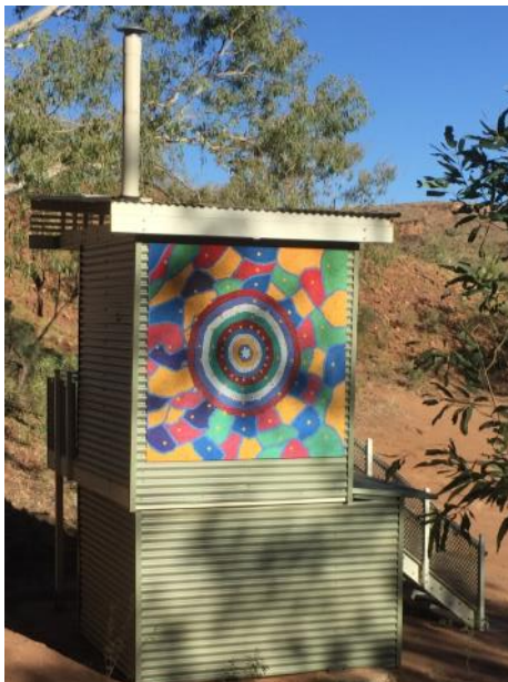
Sawpit Creek drop toilet
