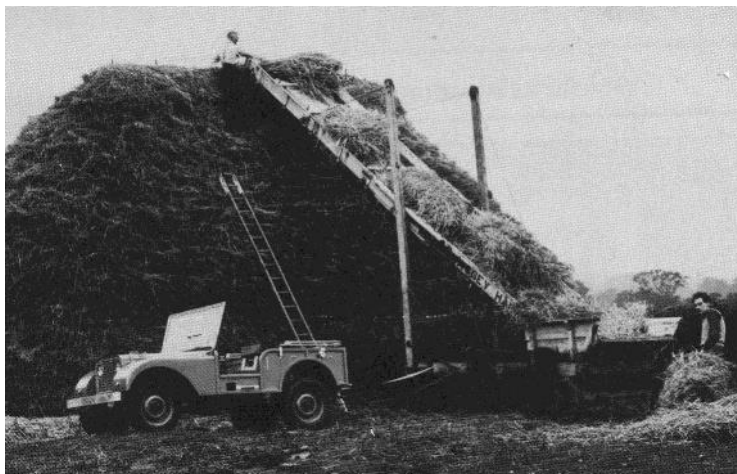
On the 15th of October 1947, the vehicle was sent to work. Here it is driving a Massey-Harris conveyor from its PTO
